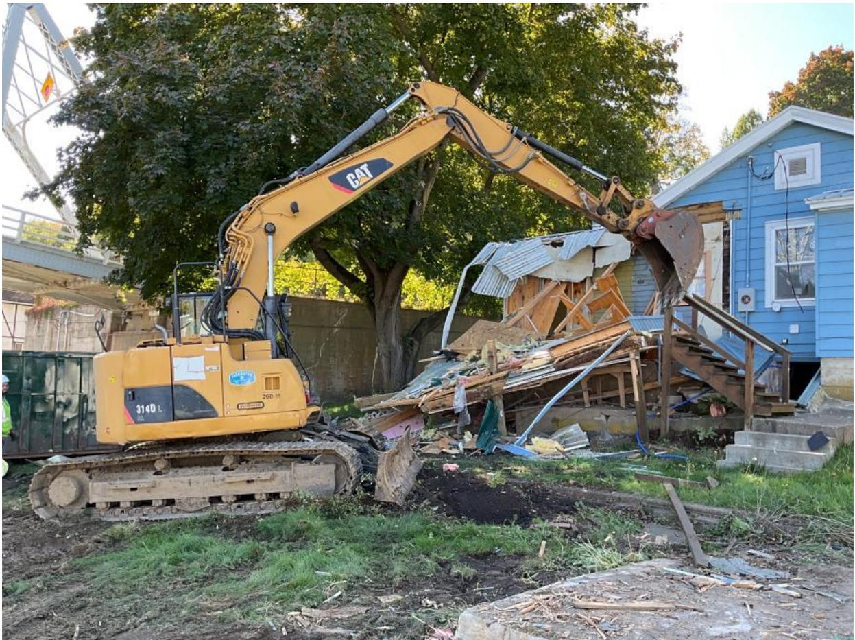
Roughly 10,000 cu. yds. of dirt and sand will be moved during construction. Heavy equipment being used will include excavators, skid loaders and lifts.
