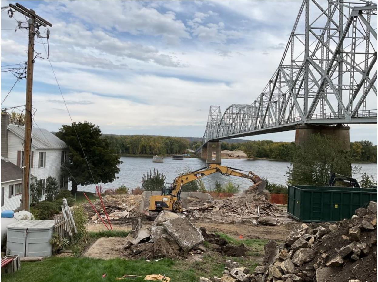
Known originally as the Black Hawk Bridge, the structure has a narrow deck at only 21 ft., with no shoulders. This makes it problematic for drivers with mechanical issues to pull over safely. The new bridge will be wider, at 40 ft. (two 12-ft. driving lanes with 8-ft. shoulders on both sides).
